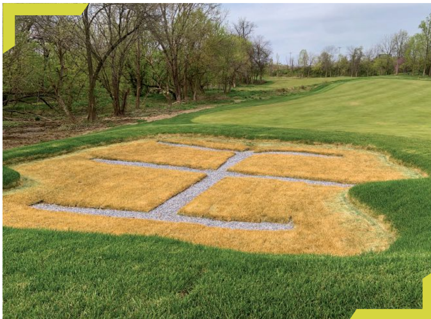
A post-herbicide treatment of a sod bunker liner during the installation process. Sod knits in before crews apply the herbicide treatment.
