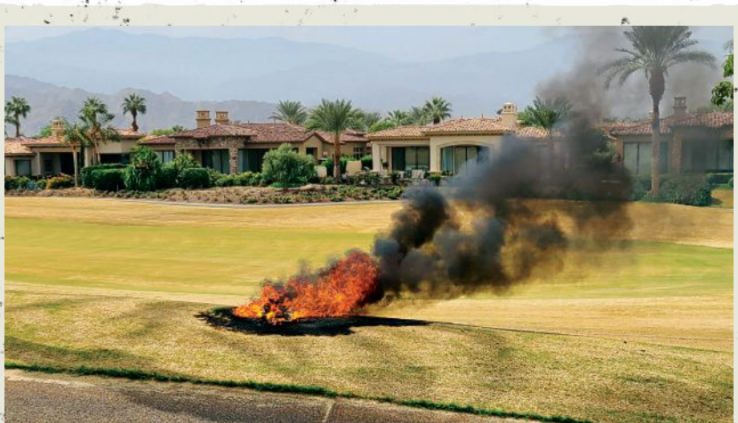
Only days away from starting their overseed, Toscana CC's irrigation system went up in smoke after an electrical surge.
