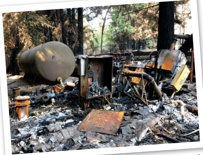
A burned-out Rain Bird pump station near Boulder Creek (Calif.) GC.
