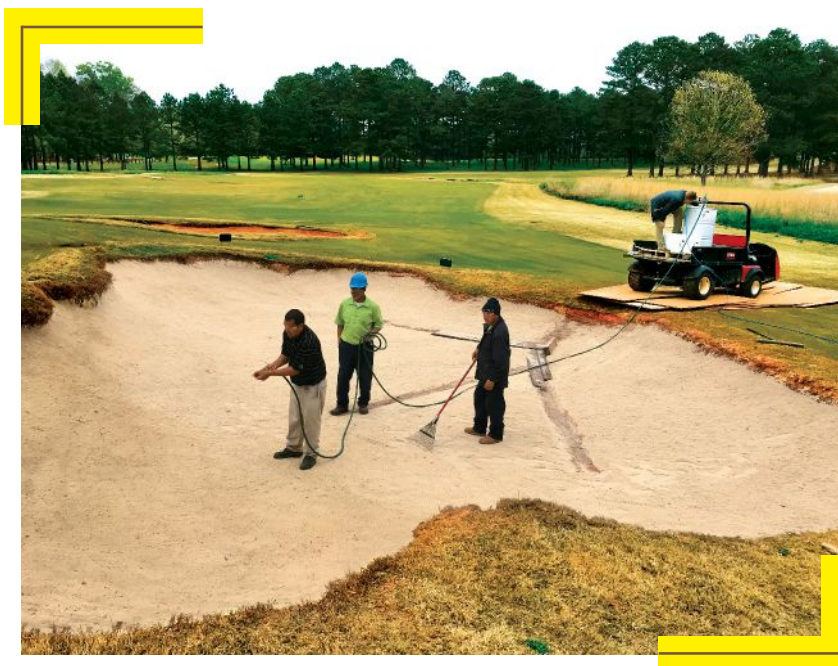
The spray-on Klingstone bunkers can be installed using a loaner pump, portable compressor and garden hose with a nozzle.
