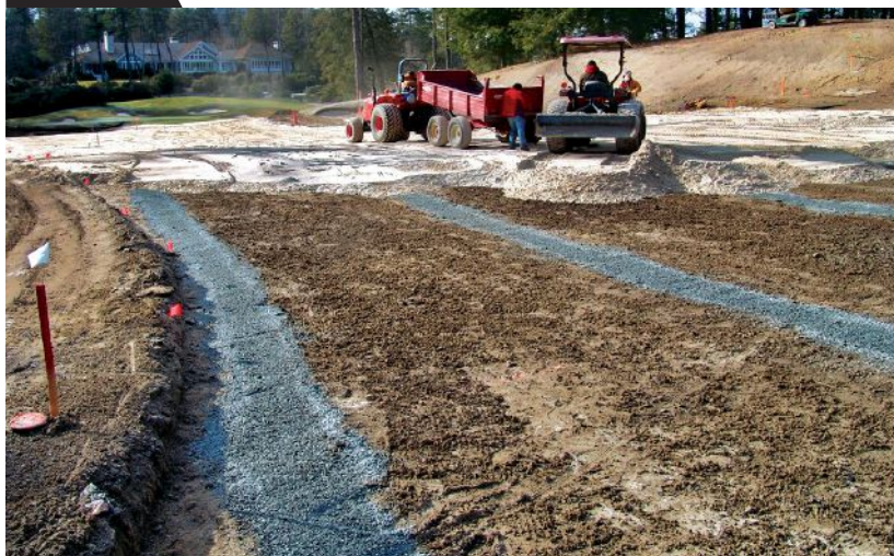
Placement of the sand cap above the soil.
