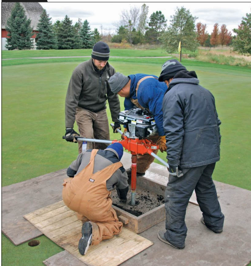
A five-inch auger bit being drilled three feet deep by staff at Medina (Minn.) G&CC to promote water infiltration in swales on native soil greens with no drainage. Channels are back-filled with pea gravel.
