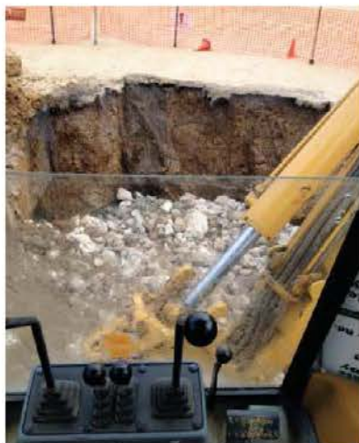
(L) To stabilize the sinkhole, the Annbriar crew dug 16 feet down and filled the hole with 200 tons of riprap. (R) The hole after it was filled and before grading.
