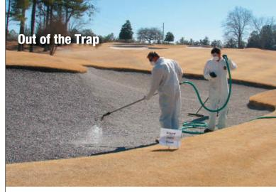
Better Billy Bunker worked with Dow to formulate a sprayable polymer that binds the gravel together, eliminating the need for a liner.
