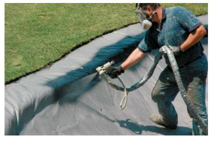
Bunker Solution combines the properties of mat and soil-binding type liners.
