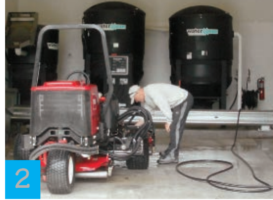
1 The turfgrass management center is comprised of two buildings, totaling 18,500 square feet. 2 The WaterStax system separates clippings and solids from water. 3 There is much more space in the new maintenance facility for equipment and employees.
