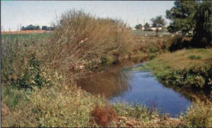
Soil-bioengineering after three years provides riparian cover and hides a rock toe.
