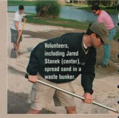
greenside bunkers that were submerged in water for nearly two weeks. The volunteers removed the old sand, repaired the drainage and added new sand.
