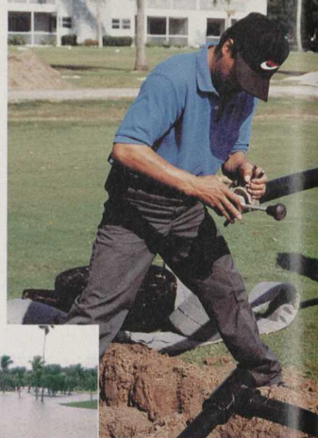
When the Seminole Golf Club flooded a few years ago, it installed a siphon drainage system from Turf Drainage Co.
