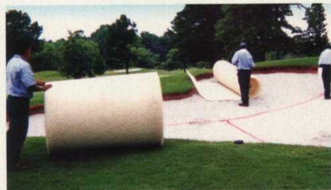
Sandtrapper for bunker renovation
