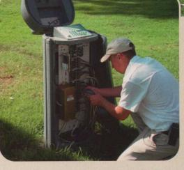
The new Signature satellites (above) easily took the place of the older outdated system. Riviera's crew members ripped out the old system and rewired the new one once it was installed (below).
