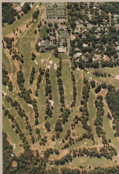
Infrared photography (right) brings irrigation system problems starkly to light.
