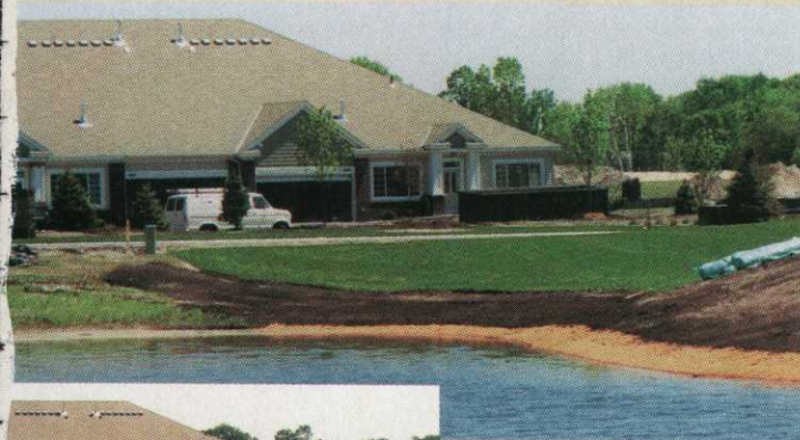
The permanent mats were installed (above) to protect the course from the waves. The healthy turf along the bank shows that the mats worked (left).
