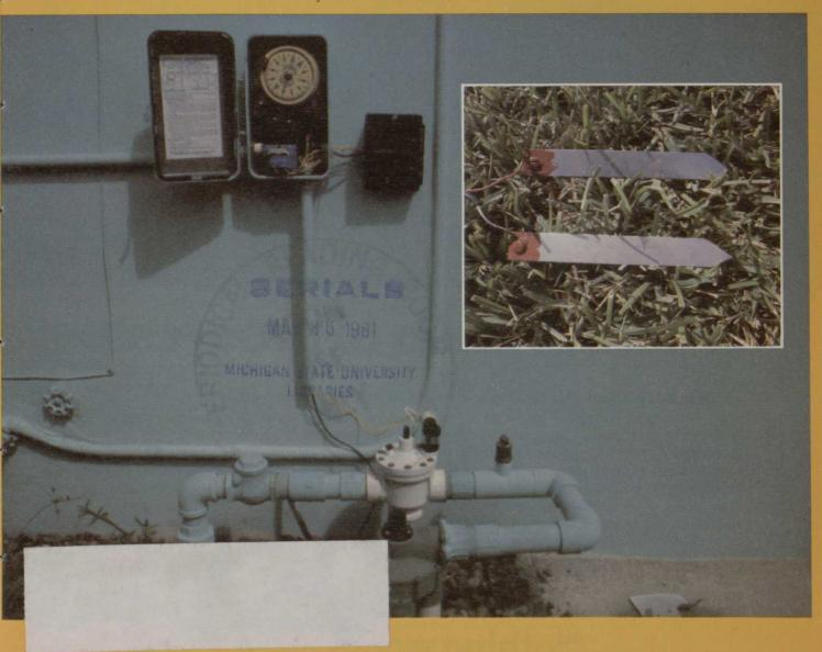
Moisture sensors for irrigation control
