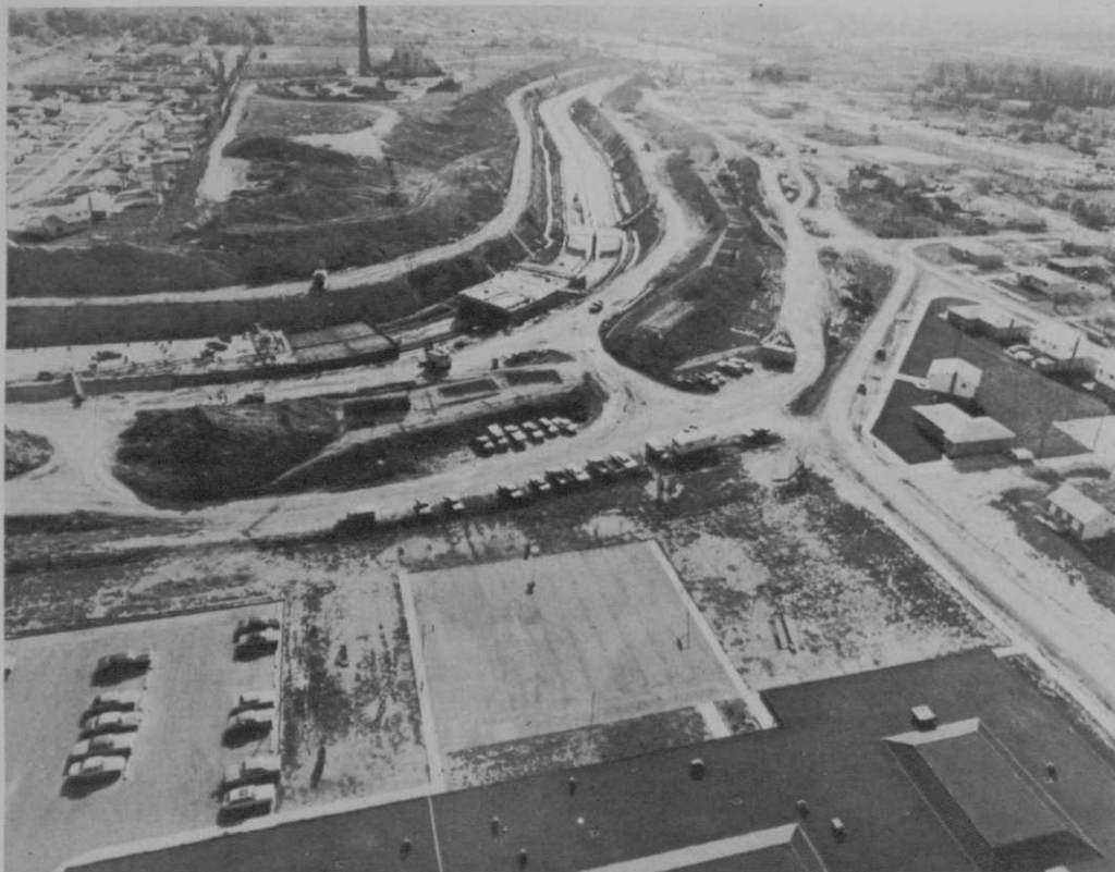
The open drain was replaced by a pollution control facility in the early '70's. Large concrete conduits are under construction and were covered following.
