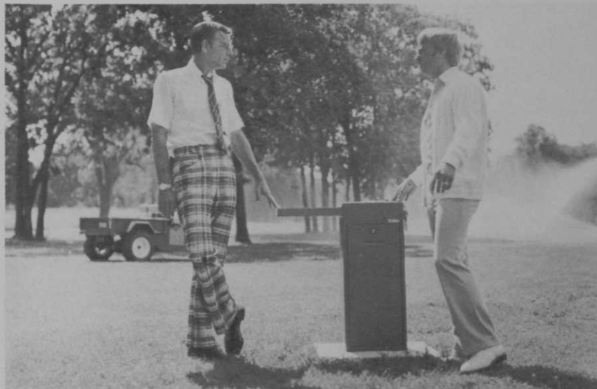
Director of Golf Jim Lucius and Superintendent Sonny Faust check one of the satellite controllers of the Southern Hills irrigation system.
