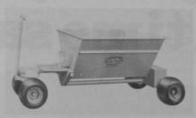
The Champion Company offers three models in its Doo-All Trailer line. Roll-Dump hoppers, available in one-cubic-yard and two-cubic-yard capacities, are also featured on two models. The third model will show the small chassis with the interchangeable flat bed in place. All units feature Terra-Tires. The two-cubic-yard chassis has a new square tongue for added strength for sharp turns under heavy load.
