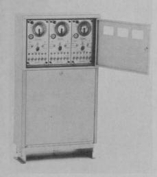
used with Moody Slave Controllers. It can stop, start or override watering programs set on remote slave controllers. Moody also makes a line of sprinklers, valves, heads, nozzles, attachments and accessories.
