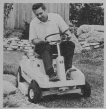
International Harvester Company offers five new finger touch control mowers in key-start or cord-start models. Each model features three-point height control. In addition, the 12hp 127 Cub Cadet lawn and garden tractor with the Sand Trap Rake, will be offered. The rake is 72 inches wide and mounted on a three-point hitch. It has a transport height of eight inches.
