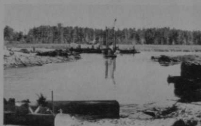
Useless swampland (above, left) was dug out and cleared with heavy machinery (left), then dredged (above) to form an attractive and functional water hazard at the Innisbrook CC, Tarpon Springs, Fla.
