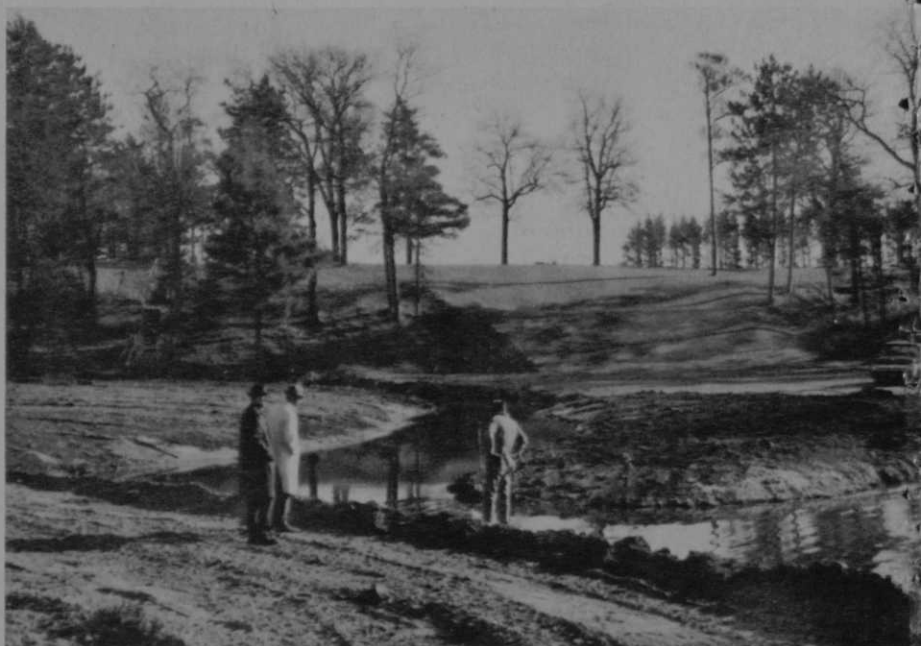
The water hazard at Stevens Point CC, Stevens Point, Wis., was improved by gently grading the embankments to provide both easy maintenance and playable lies for golfers.
