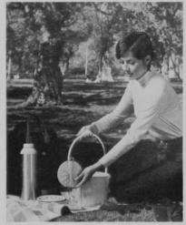
The Ogden Filter Company, Inc., offers Aquapac, a compact, portable drinking water purifier utilizing activated charcoal as a cleansing agent. The unit can be hand-pumped or gravity operated. Each sanitizing cartridge purifies 20 gallons of water. The unit weighs 10 1/2 ounces and it retails at \$19.95.
