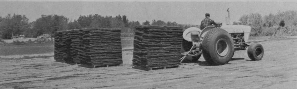
The steel skids for hauling pallettes were developed by Manuel Francis Jr.
