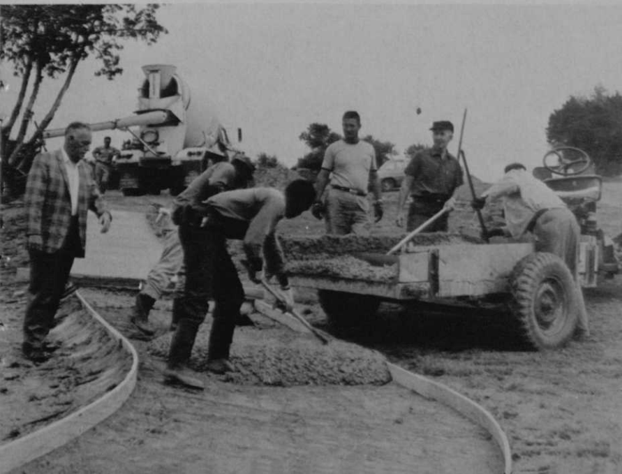
Ridgewood's Otis Beck (opposite) oversees final stages of path construction. Next step: Applying wet burlap material to implement curving. Turn-around (far left) near Las Colinas' clubhouse is both decorative and functional and the No. 15 tee and fairway (top left) is in excellent condition because cars travel only on trails. A green path (above) blends with its surroundings and does not mar the view for the residents whose homes border Quail Creek.
