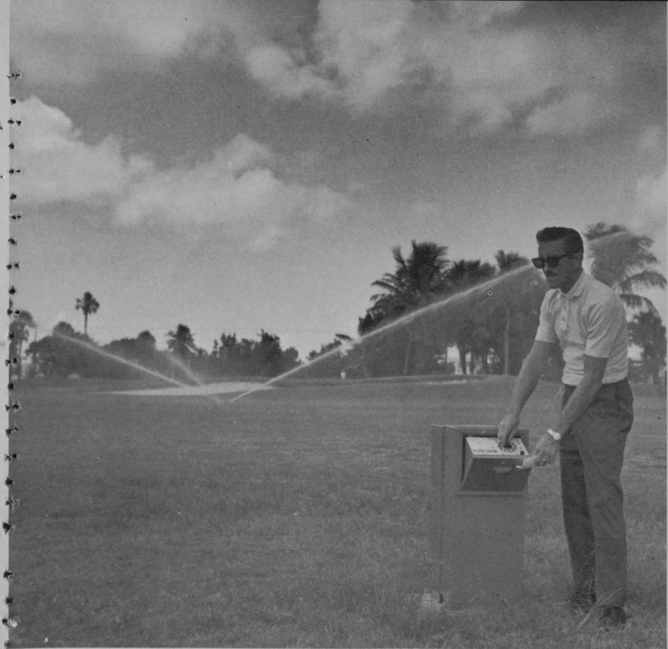
Photo at left shows how underground pipe for automatic irrigation system was laid at the Diplomat. Picture above illustrates the use of one of the many controllers that have been spotted at various zone areas. Each zone controller enables the operator to see all of the area being serviced. A central control clock is used as a master timer so that the course can have the advantages of both central and zone control.
