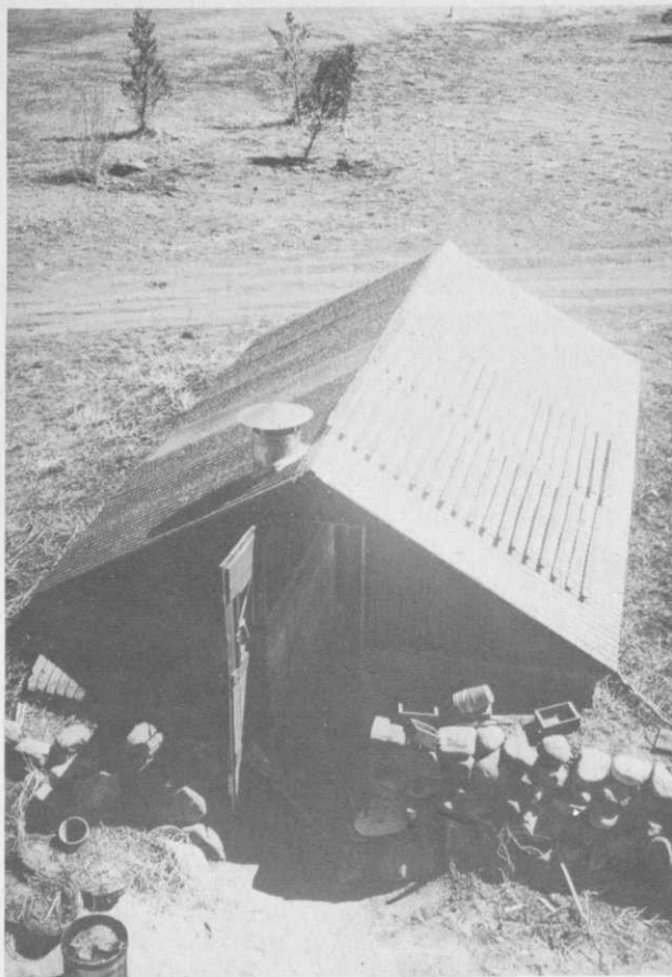
One of last year's off-season projects at Boulder CC, was building this greenhouse. The snow fence on the roof is to shade tender plants.
