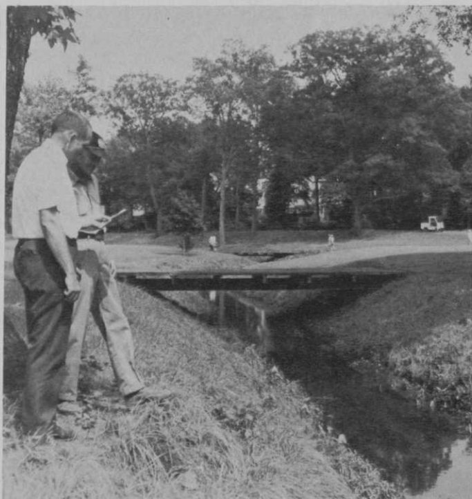
Karl Ostberg, right, and Harold Waters, SCS soil conservationist, discuss results of seeding ditch banks. Proper seeding has improved ditch's appearance.
