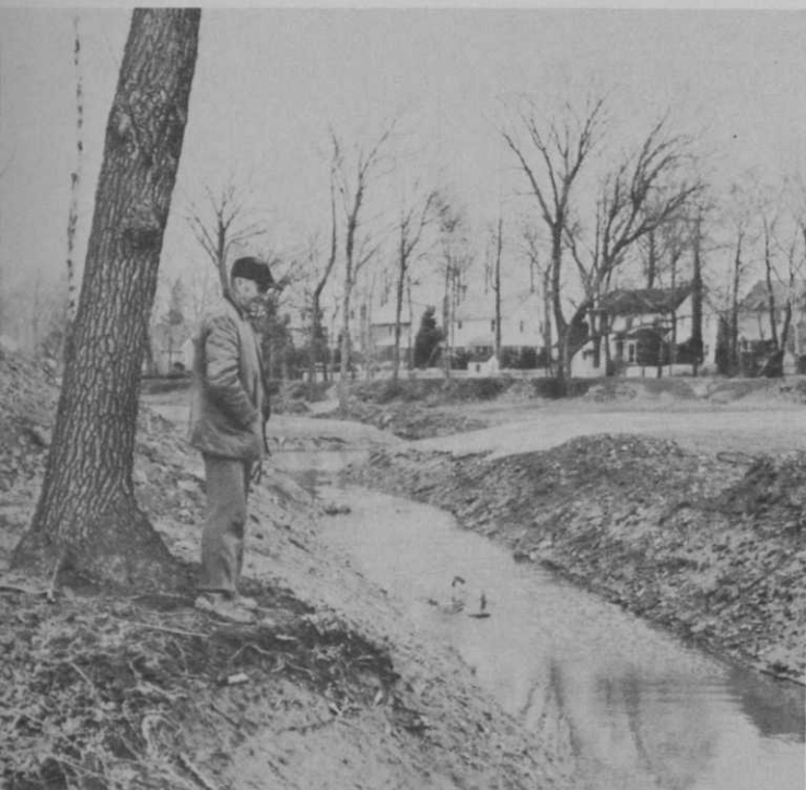
Karl Ostberg examines main drainage ditch shortly after channel improvements were made. Around 1,300 feet of the ditch were lowered and the bottom widened.
