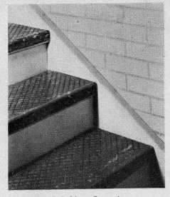
International Rubber Corp. has come out with a new Permastep heavy duty molded rubber stair tread. It is resistant to grease and oil and absorbs the noises of foot traffic.
