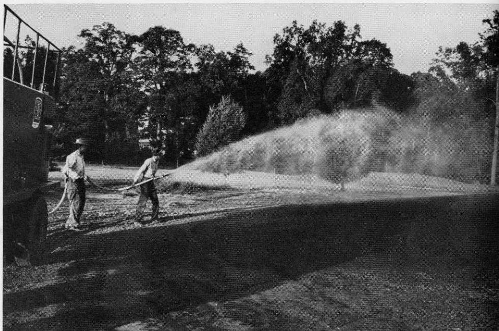
Men spray mulch and seed in water over green's surface. Job took 18 minutes on this green.
