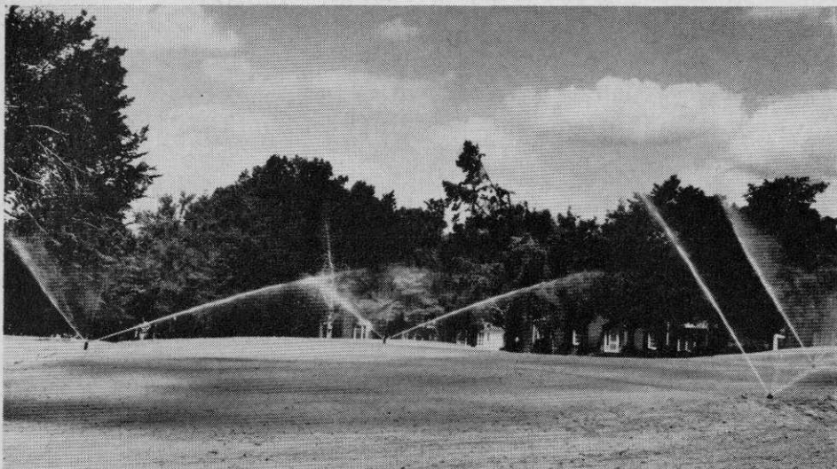
Green's sprinklers are started after mulch and seed are spread by the hydro-seeder.
