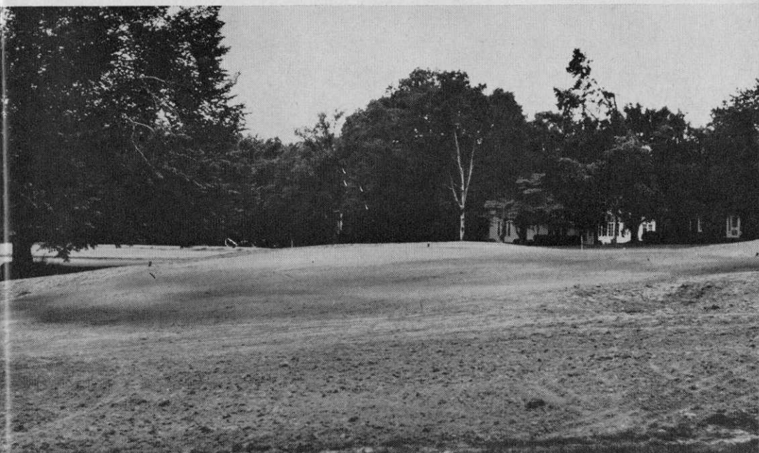
Green mulch (wood cellulose and Penncross bent seed) is shown over green after hydro-seeding
