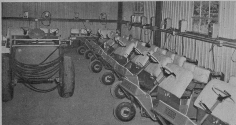
Electric cars are stored at end of new Cavalry CC maintenance building in New York.
