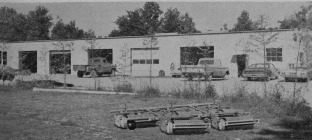
Large doors in Cavalry maintenance building lead into six separate bays of shed.
