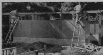
Installing main roof beam
