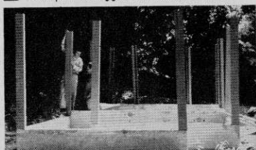
Corner posts being set in position
