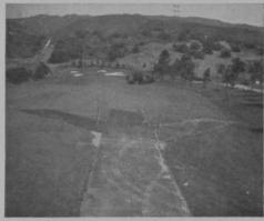
Pipes are installed in the No. 1 and No. 3 fingers and center one is left open to take the day's car traffic. On the following day, the No. 2 finger will be blocked and No. 1 or No. 3 is opened.
