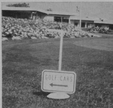
Signs installed at the bottom of a post or standard are less likely to get knocked over than those that are fastened at the top, according to Gene Stoddard, supt. at Irvine Coast CC, Newport Beach, Calif. This sign is attached to 1/2-inch angle iron that is imbedded in an old hub cap, filled with cement. It is easy to move for mowing purposes.
