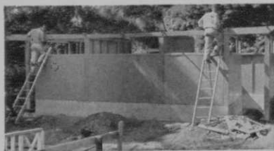
Installing main roof beam
