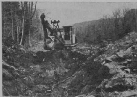
(Left) Stumping proceeds on 15th fairway. All the stumps and rocks seen here were hauled away or buried. (Right) On the 16th fairway, a backhoe opens a trench that will become burial place for stumps.
