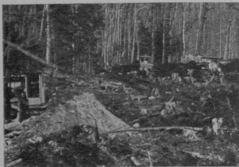
(Left) Stumping proceeds on 15th fairway. All the stumps and rocks seen here were hauled away or buried. (Right) On the 16th fairway, a backhoe opens a trench that will become burial place for stumps.
