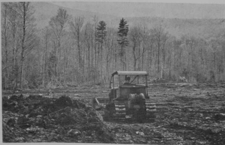
Things are beginning to shape up. Topsoil is being re-spread over the fairway that was chewed up by brush and log picker in photo at top of the page.
