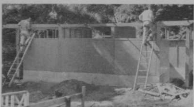
Installing main roof beam
