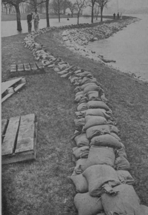
Ol' Man River keeps rolling here. Sandbags on the "low" 9 at Rock Island Arsenal delayed onset of the flood, but eventually they weren't enough, and the course was severely damaged.
