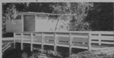
Completed and Painted Comfort Station
