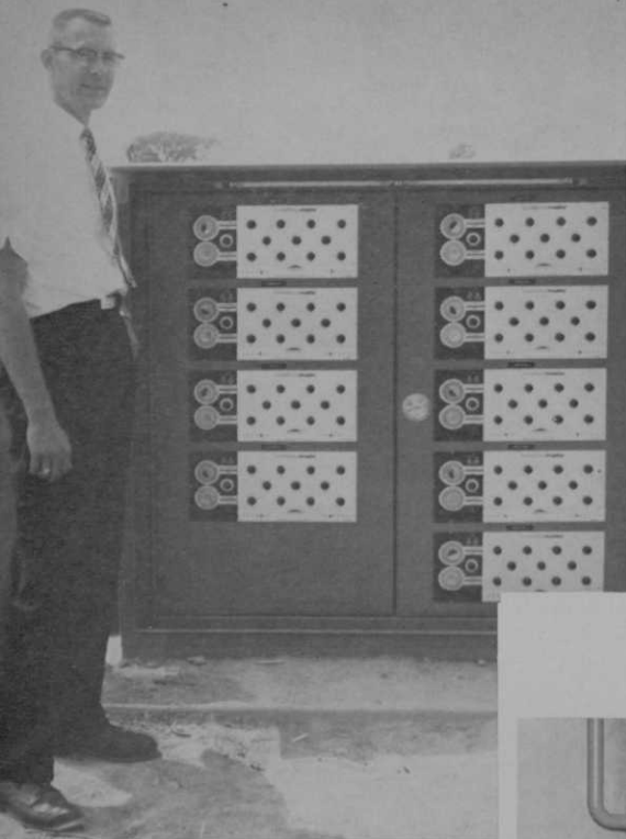
(Above) Time and sequencing controls for 99 valves in a typical course installation. Control panel is usually set to regulate watering during night hours. (Right) Up to 1,500 gpm can be pumped to many points over course area from a 16-acre water storage pond.
