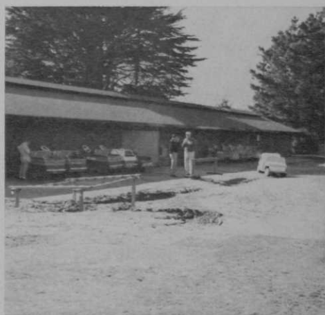
New car storage room and caddie house are being used as temporary clubhouse during reconstruction.
