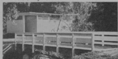
Completed and Painted Comfort Station
