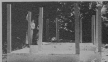
Corner posts being set in position
