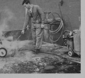
wash rack where much of our equipment is washed and, if necessary, can be wiped dry. A grease pit is also located here. It measures 16-feet long by 3-feet wide and 6-feet deep, with descending steps. This makes it possible to service practically every piece of equipment owned by the club. A grease pit and car wash makes it easy to keep up with regular oil changes, chassis lubrication and cleaning in all types of weather.
