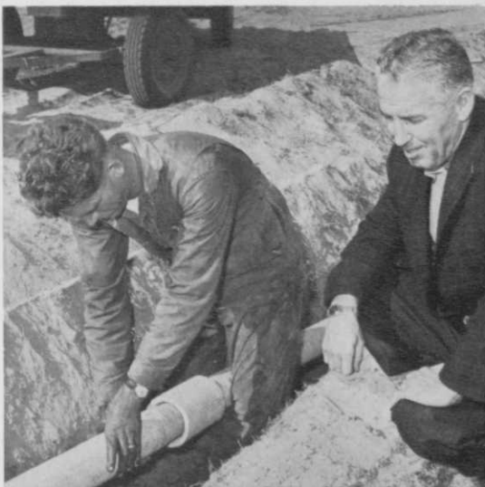
Bob Baldock is seen in both photos as he inspects the installation of irrigation pipe at the Shore course. At left, a joint is being welded with a solvent. At right, a connection is made by inserting lengths into a coupling. A rubber gasket and lubricant are used in making the connection water tight.
