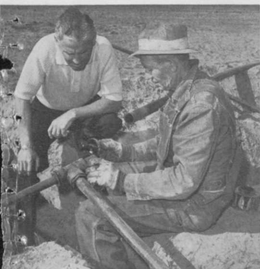
Bob Baldock is seen in both photos as he inspects the installation of irrigation pipe at the Shore course. At left, a joint is being welded with a solvent. At right, a connection is made by inserting lengths into a coupling. A rubber gasket and lubricant are used in making the connection water tight.
