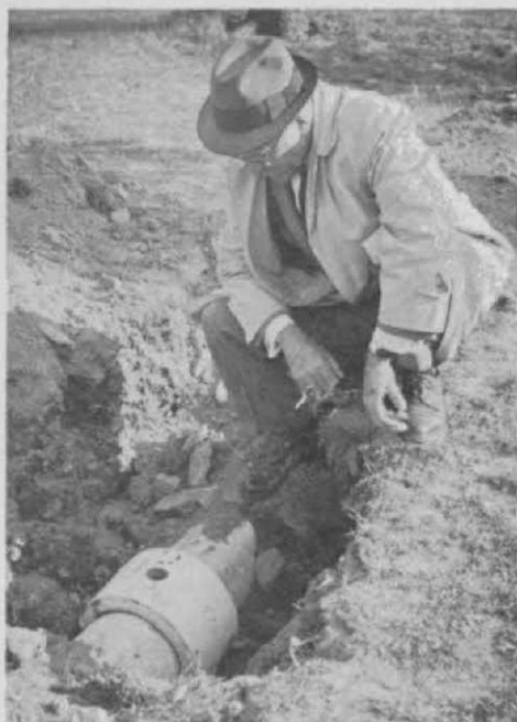
Ed Hennessy of K & M looks over a pre-tapped coupling, which simplifies installation of risers and snap valves.
