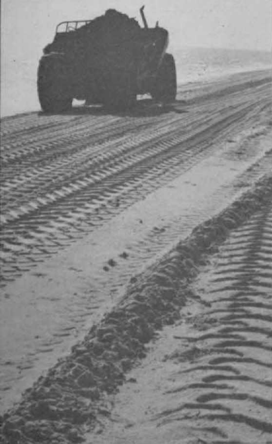
Earth mover hauls tons of silt from Alligator Lake more than one mile to Isle Dauphine course. At high tide machine often ran with one wheel in the Gulf of Mexico.
