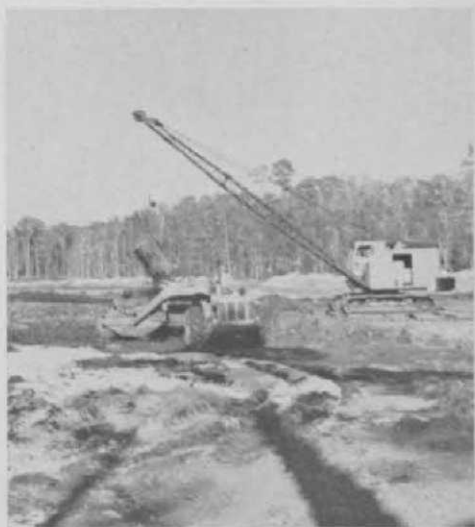
Digging silt from bottom of Alligator Lake to be used as topsoil on the course. Lake was pumped dry by Maddox firm and about 30,000 yards of silt was removed.
