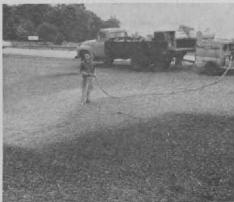
This site is getting a bath of Turfiber and asphalt emulsion for anchorage of seed in a gully.
