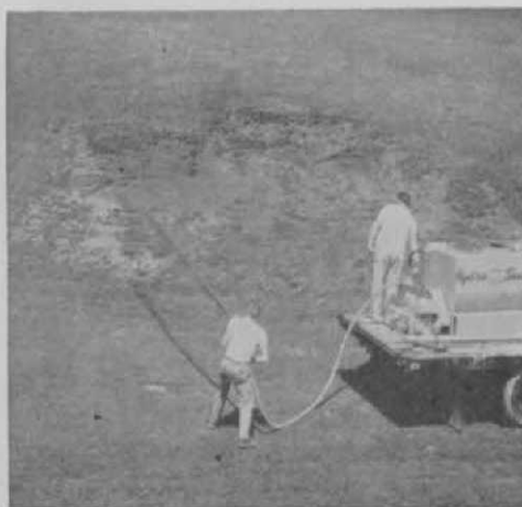
Slope on Avon Fields GC in Cincinnati is being patched with seed, fertilizer and Turfiber mixture.
