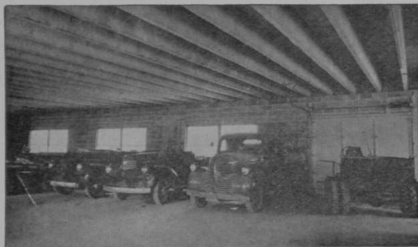
Prestressed roof slabs give column-expanse to permit greater freedom of movement for vehicles within the building at Butterfield CC.
