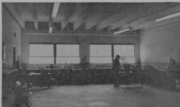
Prestressed roof slabs give column-expanse to permit greater freedom of movement for vehicles within the building at Butterfield CC.
