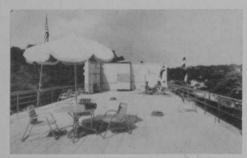
able areas, such as for recreation, sunbathing, etc. The tile also serves to keep roofs from deteriorating. Light gray in color, the tile is highly reflective, thereby minimizing heat absorption. Called Promenade Tile, the new K & M product is installed by trowel on a cold asphalt cement base in an operation similar to installing interior plastic tile. Standard size is 12 x 12 ins. and half tile, 12 x 6. Both are 5/16 ins. thick.
